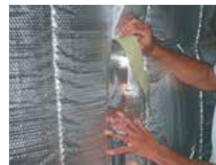
Overlap alumaflex by 100mm and use alumaflex tape on the sidelaps.
