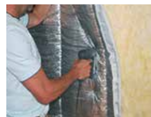
Staple alumaflex vertically to the studwork.
