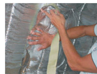
Overlap alumaflex by 100mm and tape the laps.
