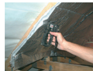
Staple alumaflex to the underside of the rafter.
