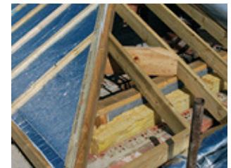
Staple alumaflex over the rafter.
