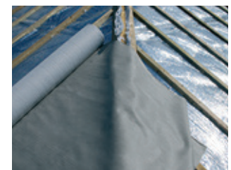
Fit breathable membrane over battens and alumaflex.
